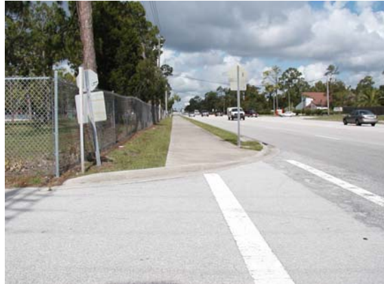
Looking west along Taylor Road – the school entrance crosswalk and curb ramp should align with the sidewalk
